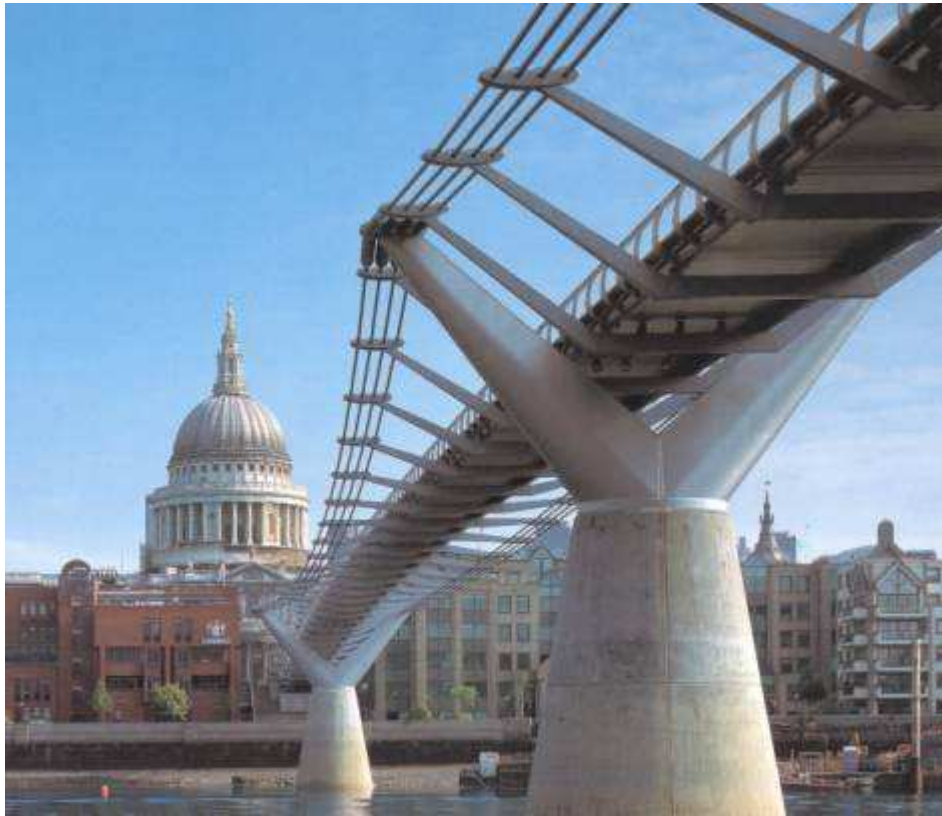
Figure 3 Centre span of the Millennium Bridge
